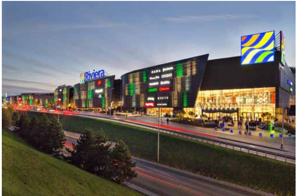
Riviera Center in Gdynia/Press material by Maryland real Estate
